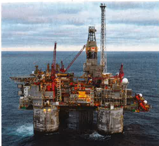
The Heidrun tension leg platform (TLP) in the North Sea was commissioned by Conoco in 1995 as the world's fifth TLP and is the only one to be built using reinforced concrete. Operated today by Equinor, the platform is connected to 51 producing wells in water depths of more than 1,100 ft. Source: Equinor/Harald Pettersen.
